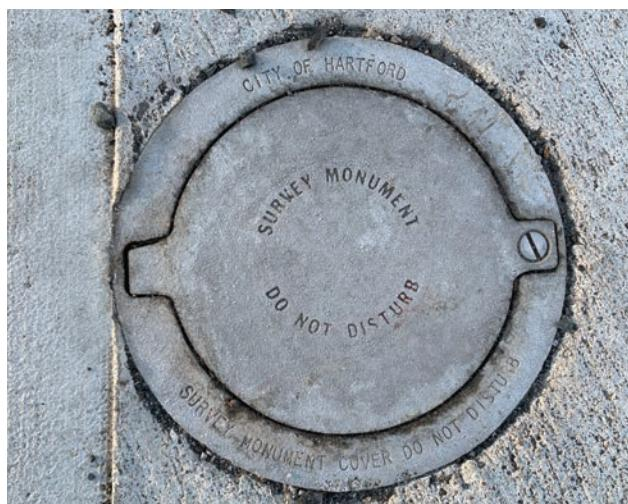
This metal cover marks the location of a monument that is now covered by a newly built sidewalk. Using a screwdriver, a surveyor would be able to uncap this monument in order to conduct an accurate property survey of this Hartford city block. The cap warns passersby, "Do Not Disturb." According to Connecticut General Statute Section 47-34a, "disturbing" a monument carries a fine of at least \$500. photo: Arianna Basche and Mitch Curry
